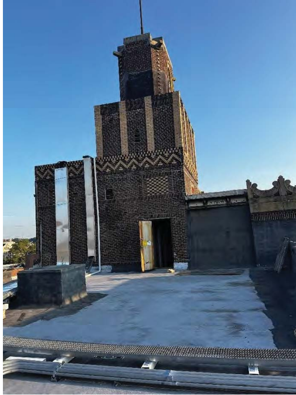
Photograph 9 - Rooftop structures with roofing membrane.
