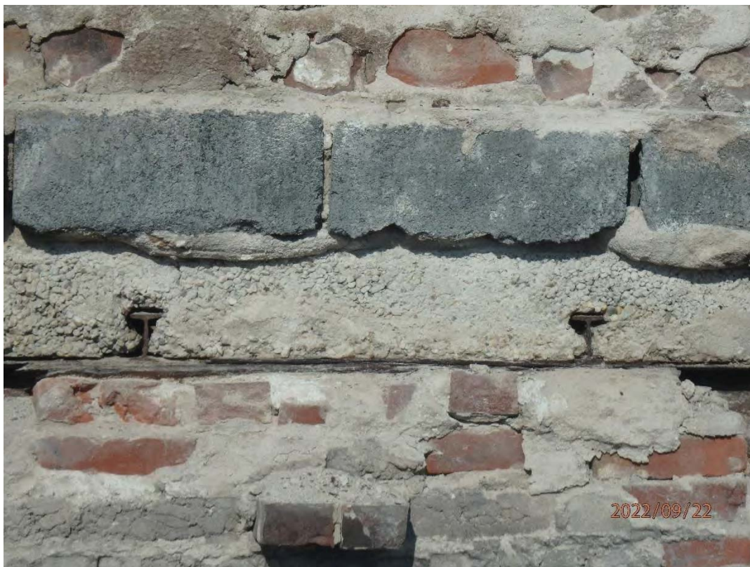
Photograph 7 - Steel framing with concrete slab.
